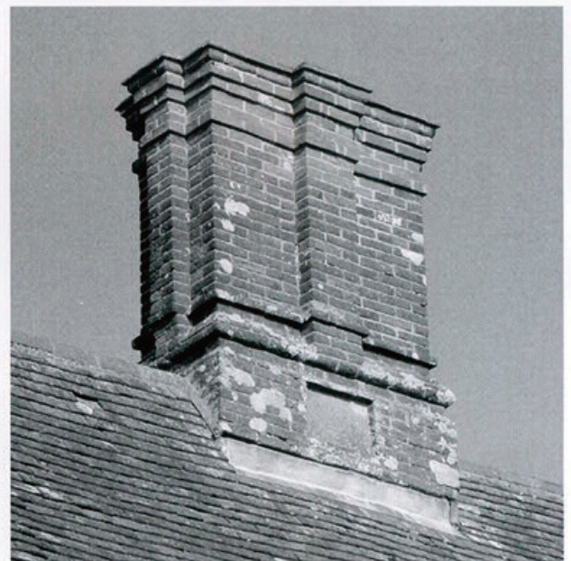
Fig. 10: 17thC brick chimney stack
