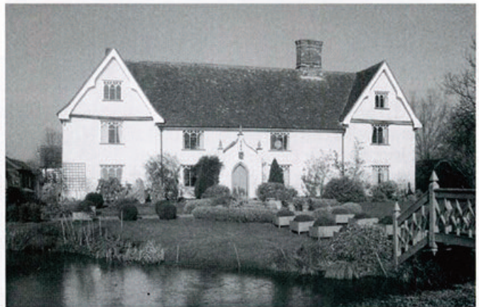
Fig. 11: Bedfield Hall, South side
