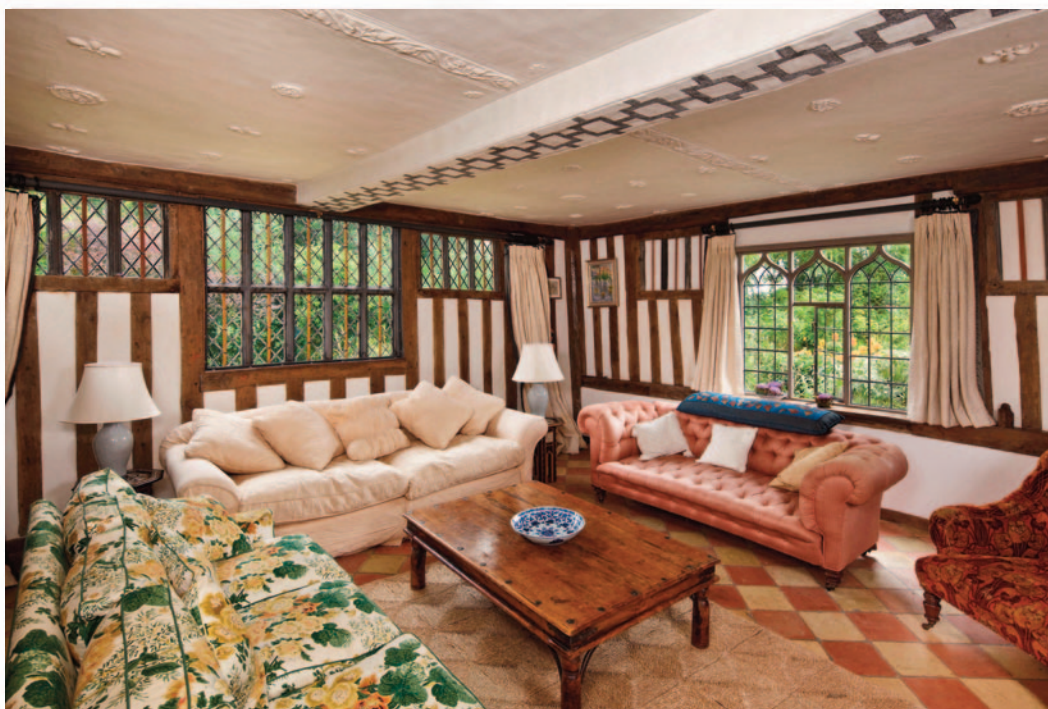
Fig. 4: The parlour, 1630. Note the closer proximity between the plastered bridging beam and the underside of window opening. Close stud work originally covered and 'wind sealed.'
