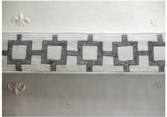
Fig. 5: The parlour, a section of the restored carbon-painted design; approximately 65% is original.
