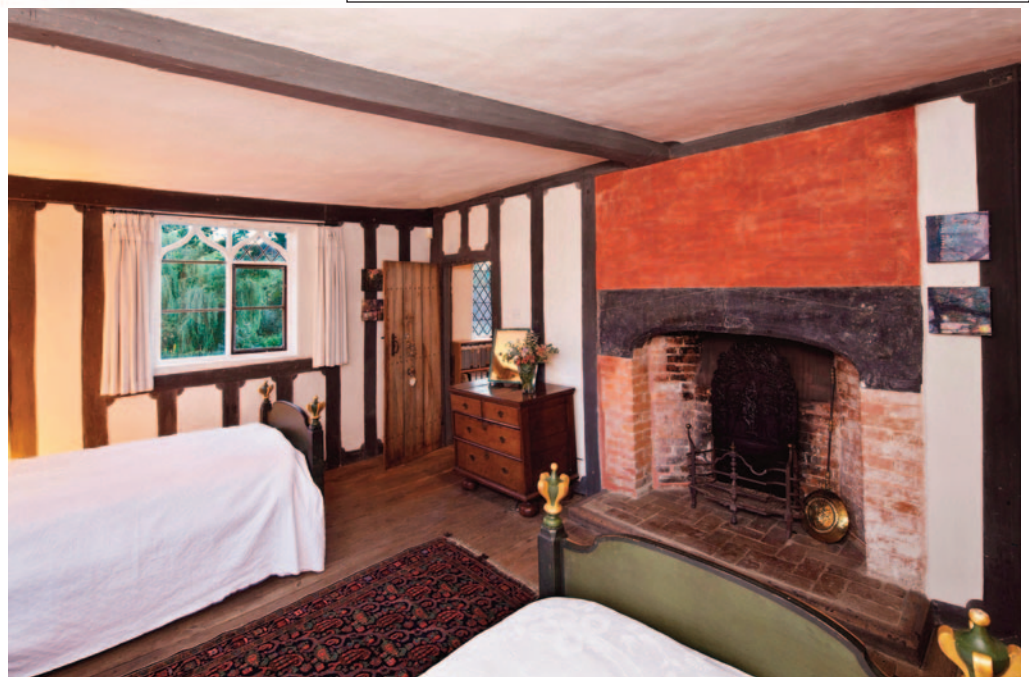
Fig. 10: Kitchen chamber 1620. The painted studs with additions make rudimentary columns, adjacent to the painted hearth. Faux 'Belgium black' on the arch imitates marble and the red paint above over the squared-up plaster imitates terracotta tiles.
