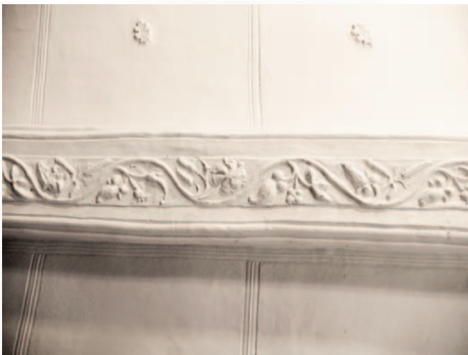
Fig. 1: Parlour chamber, 1630: detail of the unpainted mouldings on the underside of the plastered bridging beam.
