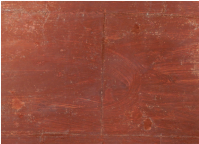
Fig. 12: Kitchen chamber. Wide brush marks shows the speed the painter needed to work on barely dried plaster.
